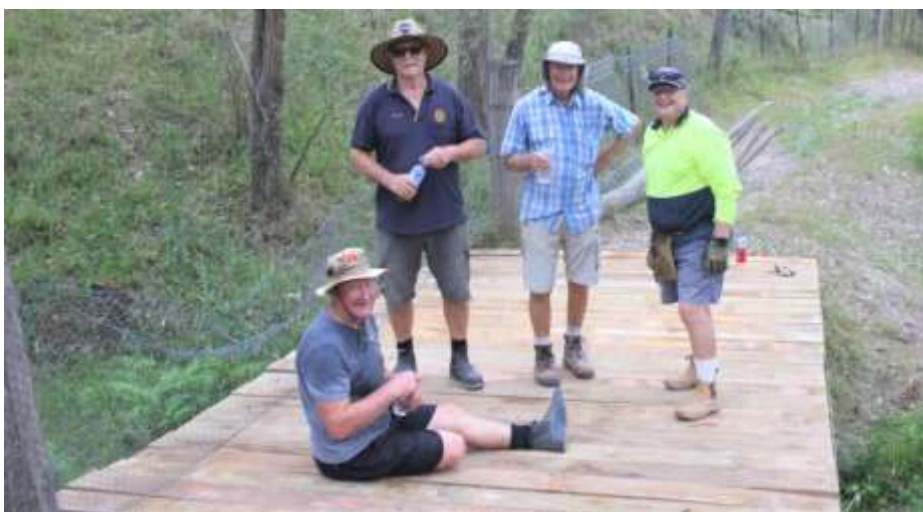
Bridge repair at Hawkesbury High School.....
